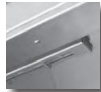
Stainless Steel Thermal Breaker (Interior)
