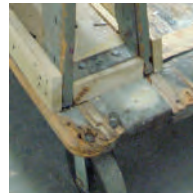
Wood—splinters and rot
